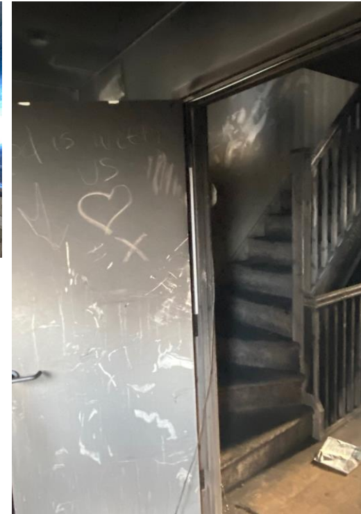
Kitchen Fire Door Removed Closer – Smoke Damage
